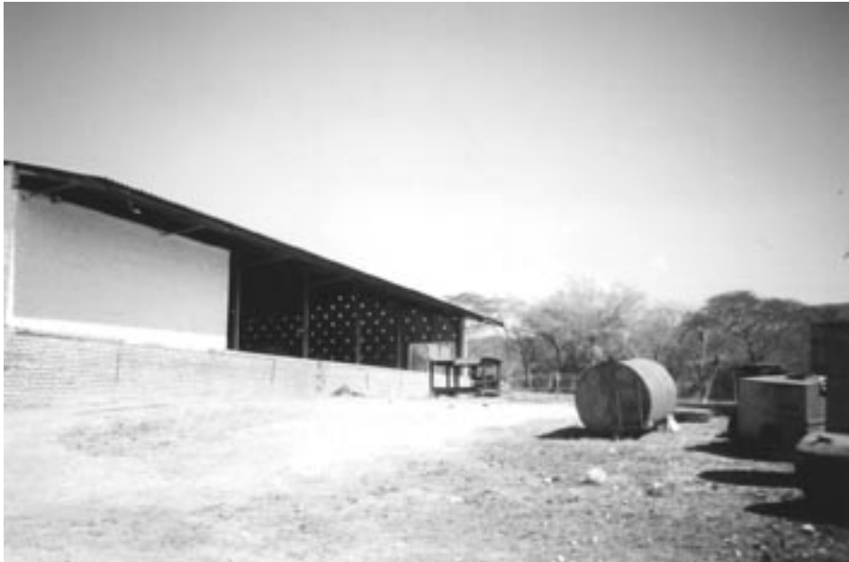
A deserted packing shed after the handover: the Amm farm, Letsitele.
